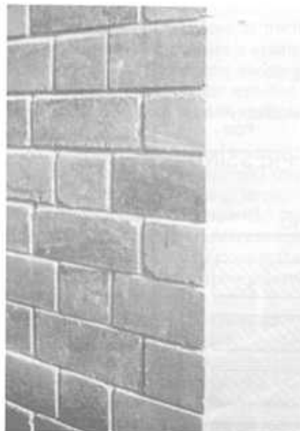
Coordination of the block dimensions to achieve a proper bond
