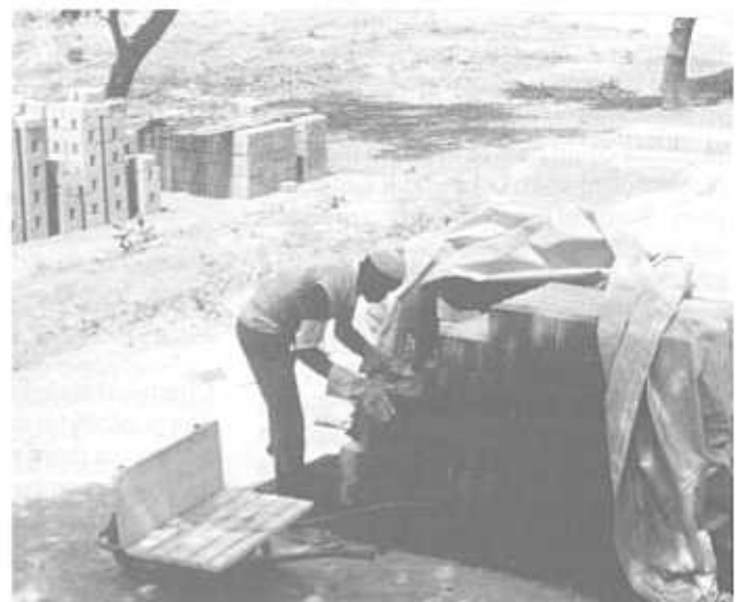
Curing under a plastic film
