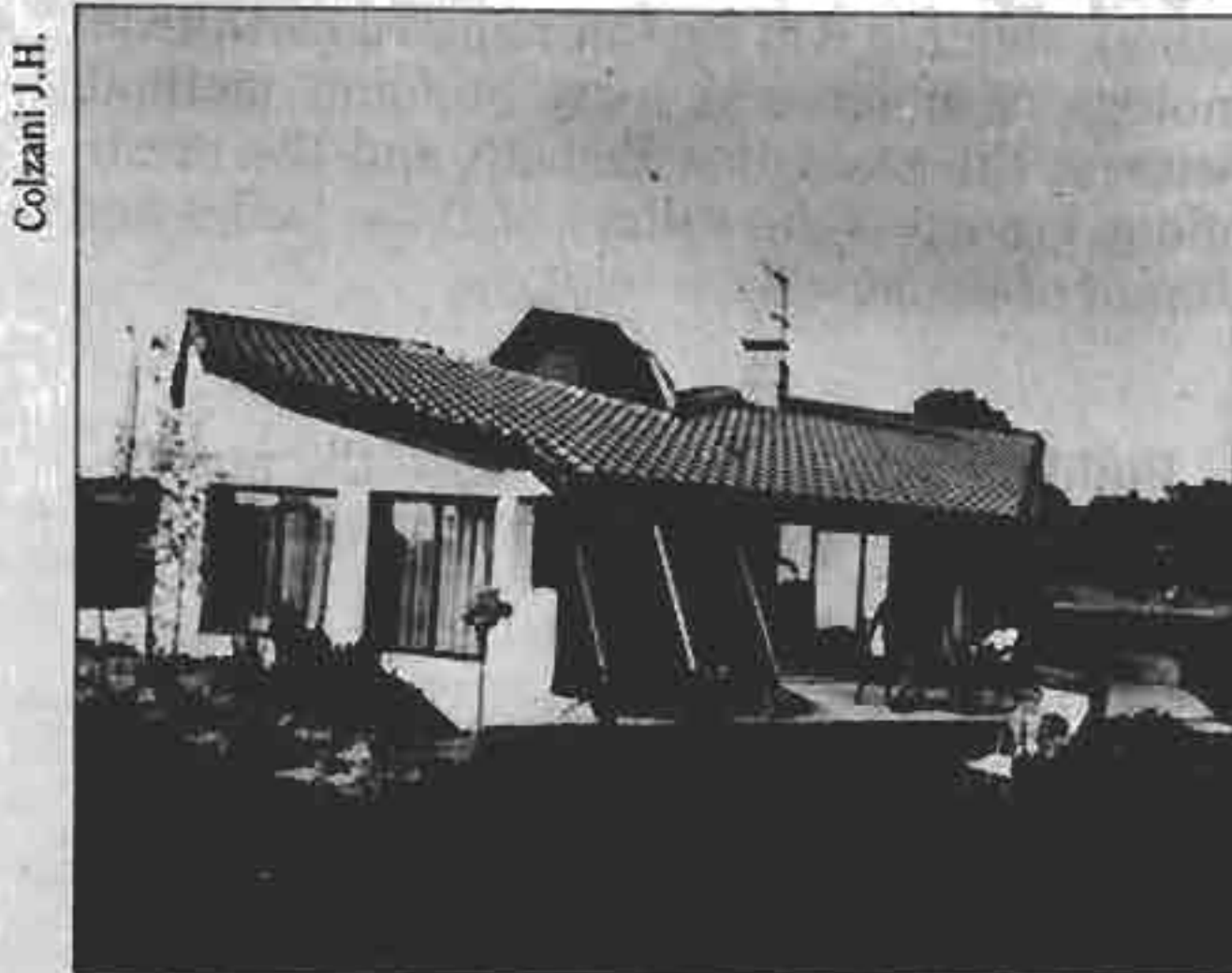
FIGURE 338: "SOFT HOUSE". SOLAR HOUSE BUILT BY COLZANI J.H. OF THE ARCHECO GROUP OF TOULOUSE. THE HEAT RETAINING INTERIOR WALLS ARE IN STABILIZED EARTH WALLS.
