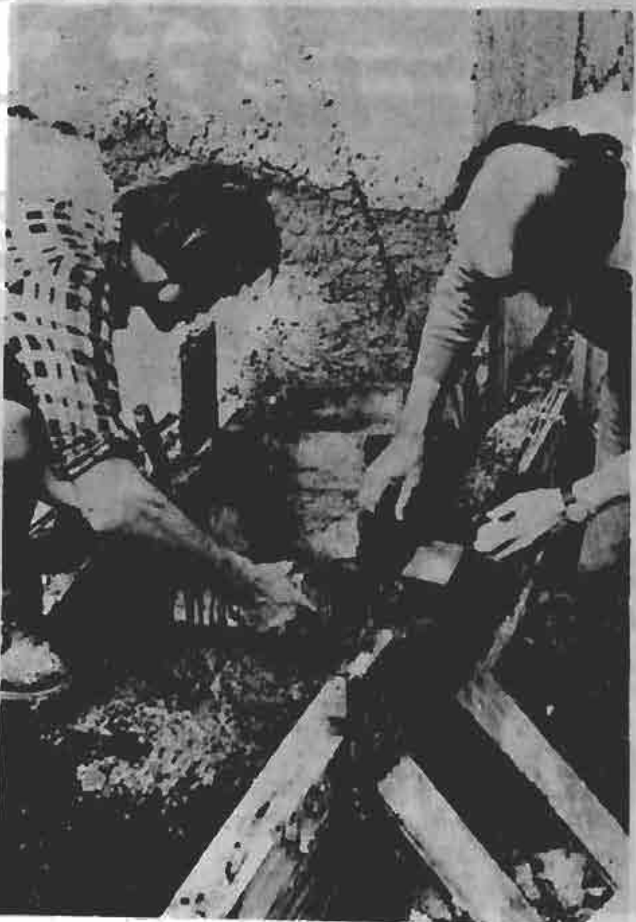
FIGURE 311: LAYING THE FIRST BRICKS OF THE FOOTING
