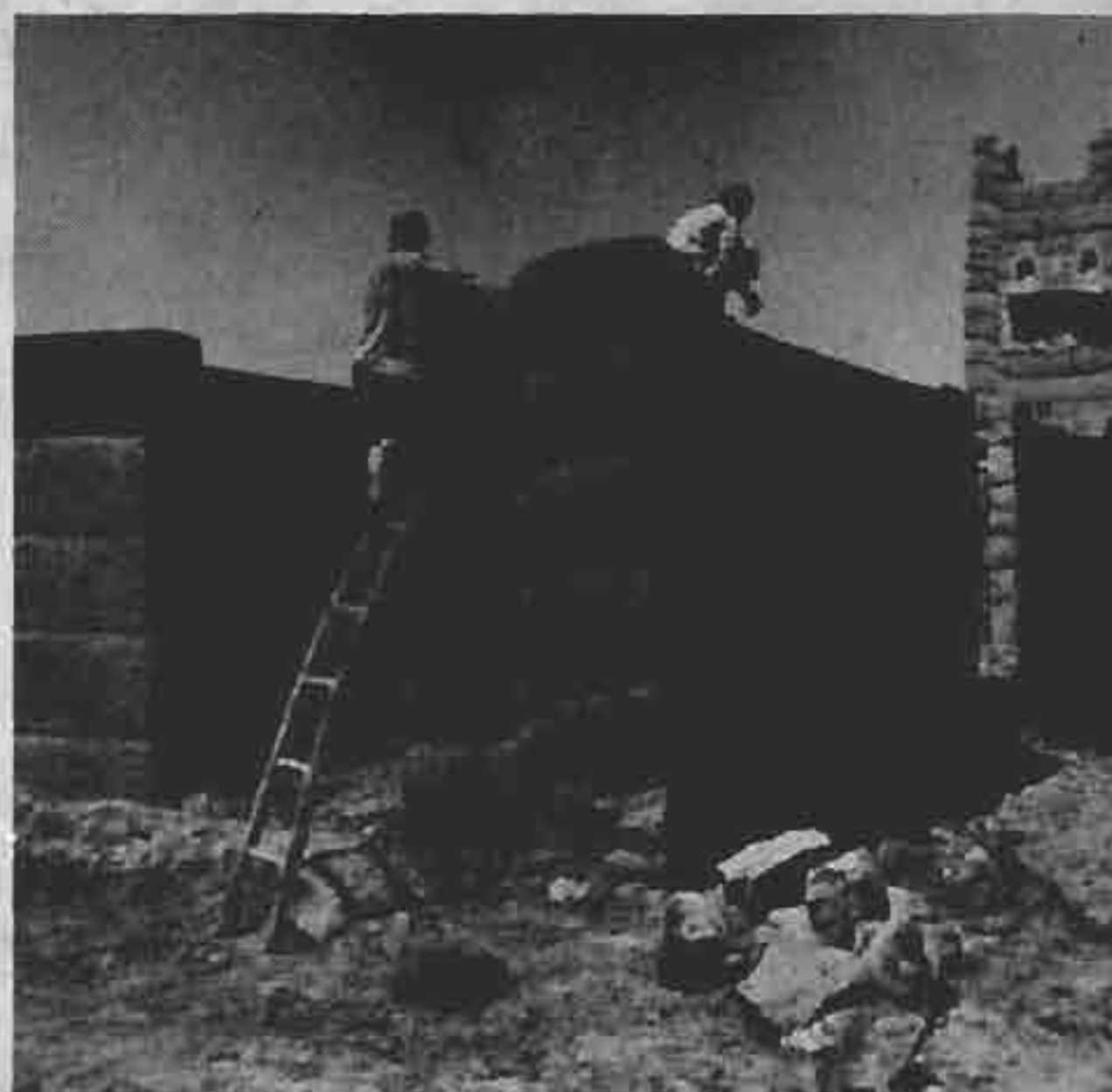
FIGURES 138/138A: MASONS SHAPING A HUGE MUD "SAUSAGE" IN ITS FINAL POSITION
