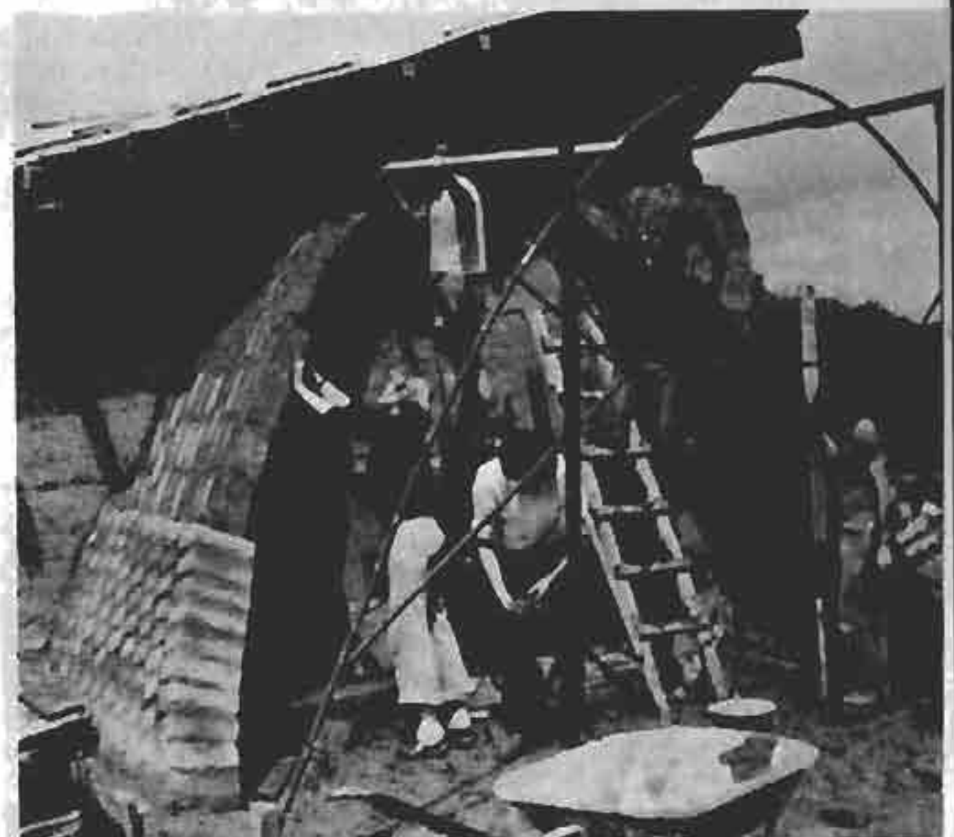
FIGURE 314: THE BUILDER ABOVE LEFT CHECKS THAT THE SHAPE OF THE VAULT REMAINS TRUE
