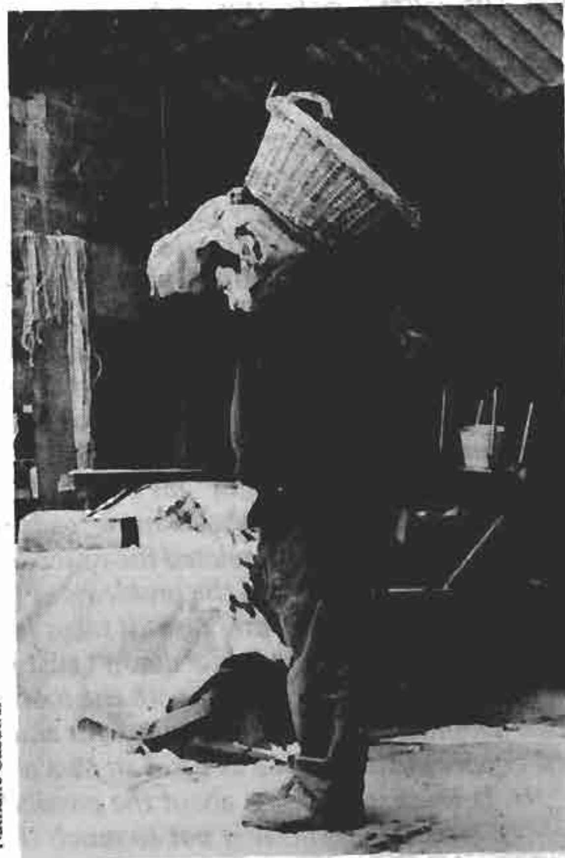
FIGURE 53: HOW THE EARTH IS CARRIED IN A WICKER BASKET
