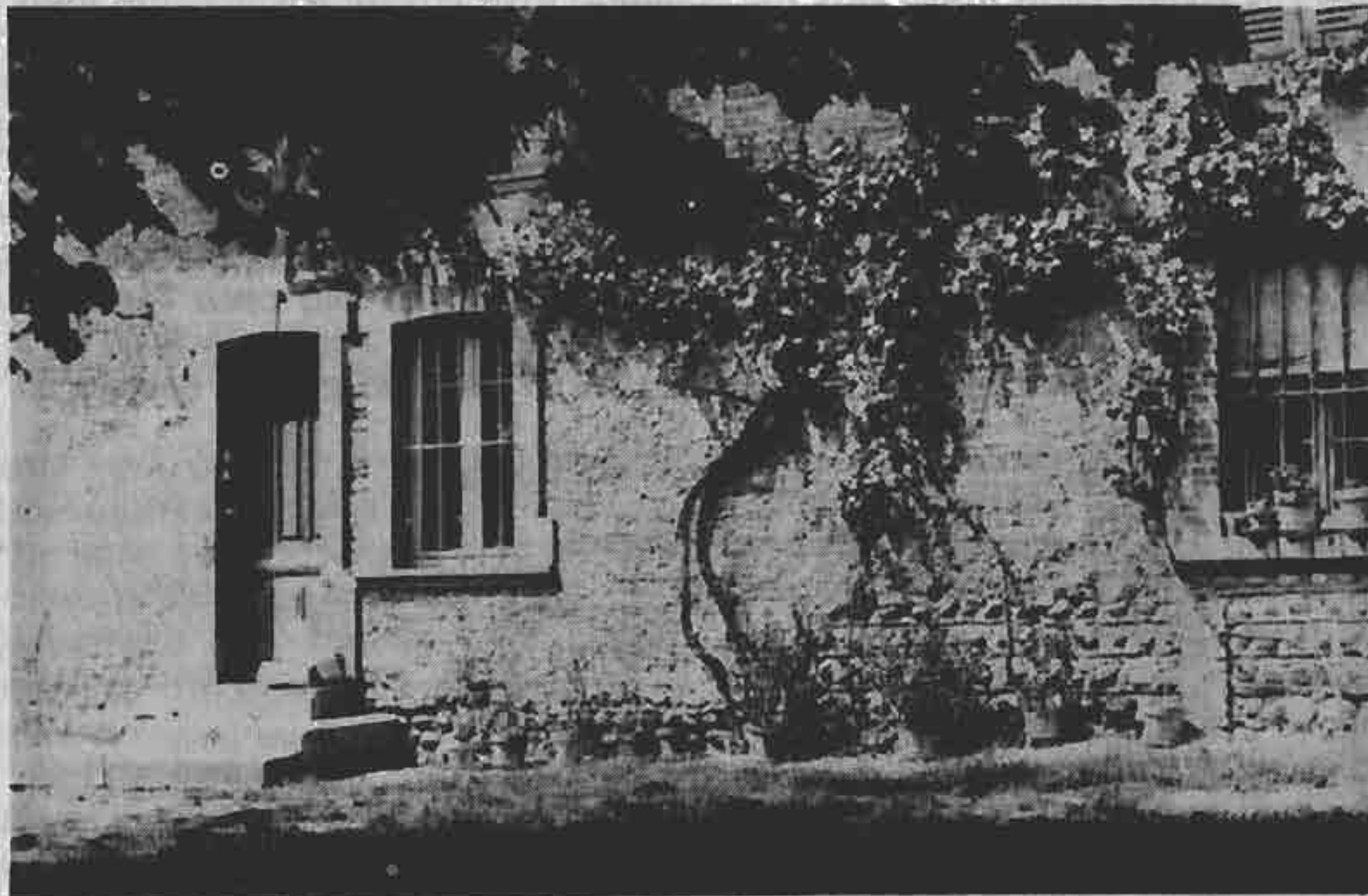
FIGURE 47: FACADE OF THE LIVING ACCOMMODATION.
