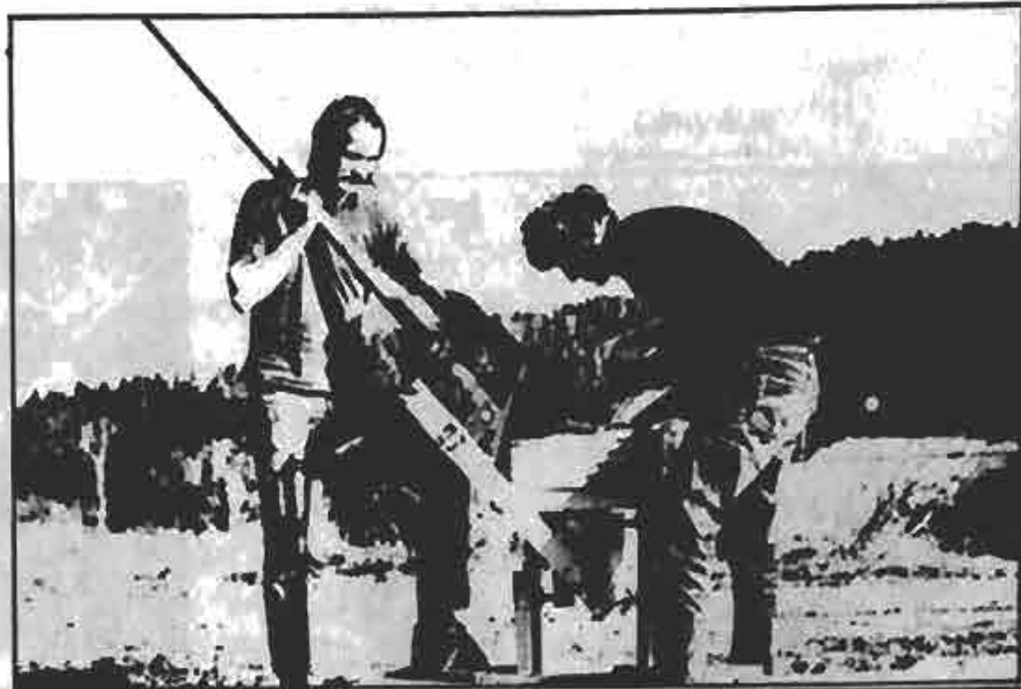
Filling the mould
