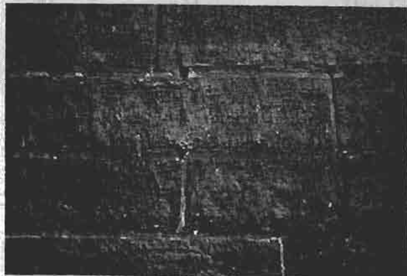
FIGURE 23: RAMMED EARTH WALL SECTIONS WITH VERTICAL JOINTS. (BRESSE, FRANCE).
