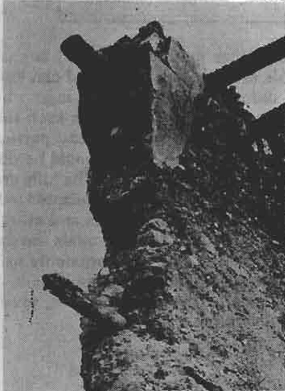
FIGURE 27: WOODEN RING-BEAM WITHIN THE RAMMED EARTH WALL
