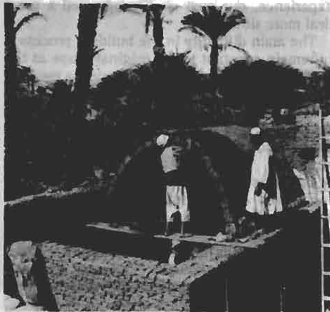
FIGURE 309: CONSTRUCTION OF NUBIAN VAULT NEAR ASWAN (EGYPT)
