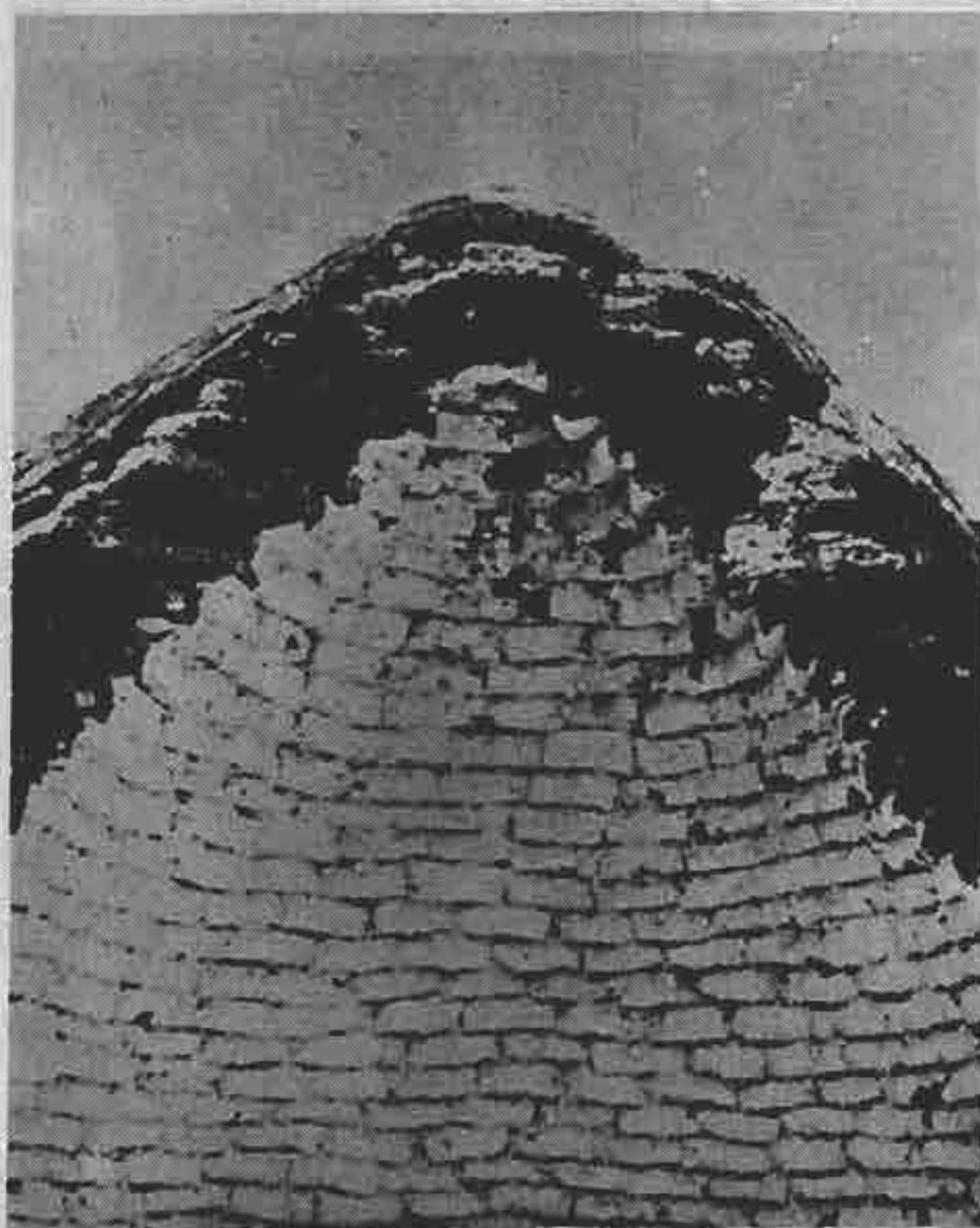
FIGURE 318: CORBEL DOME. THE BRICK PROJECTS BY APPROXIMATELY ONE TENTH OF ITS LENGTH.
