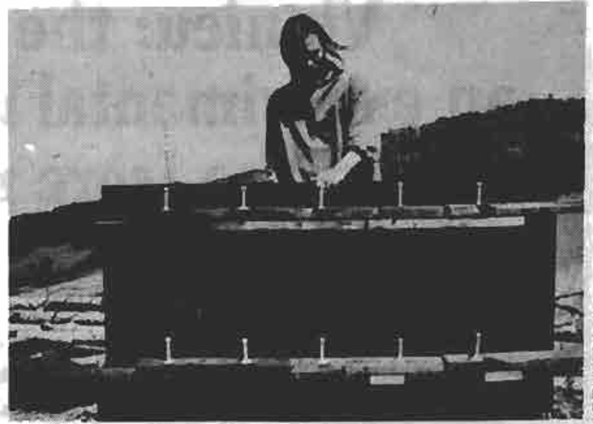
FIGURE: 97 HINGED FORMWORK ALLOWING FOR CURVED WALLS AND POSTS - HORIZONTAL POSITION (LE PIN, 1975)
