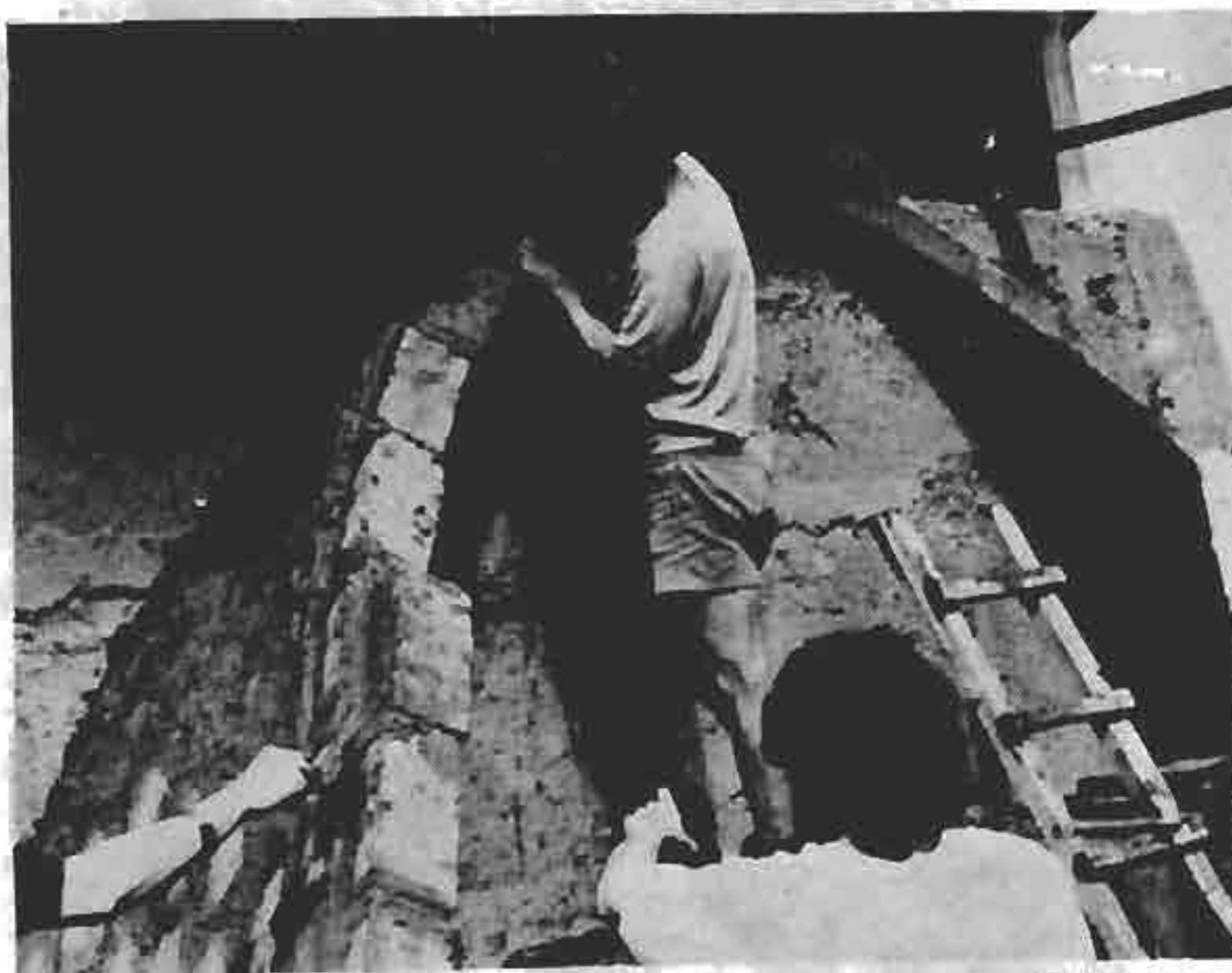
FIGURE 313: THE BRICKS AT THE APEX ARE THE MOST TRICKY TO LAY
