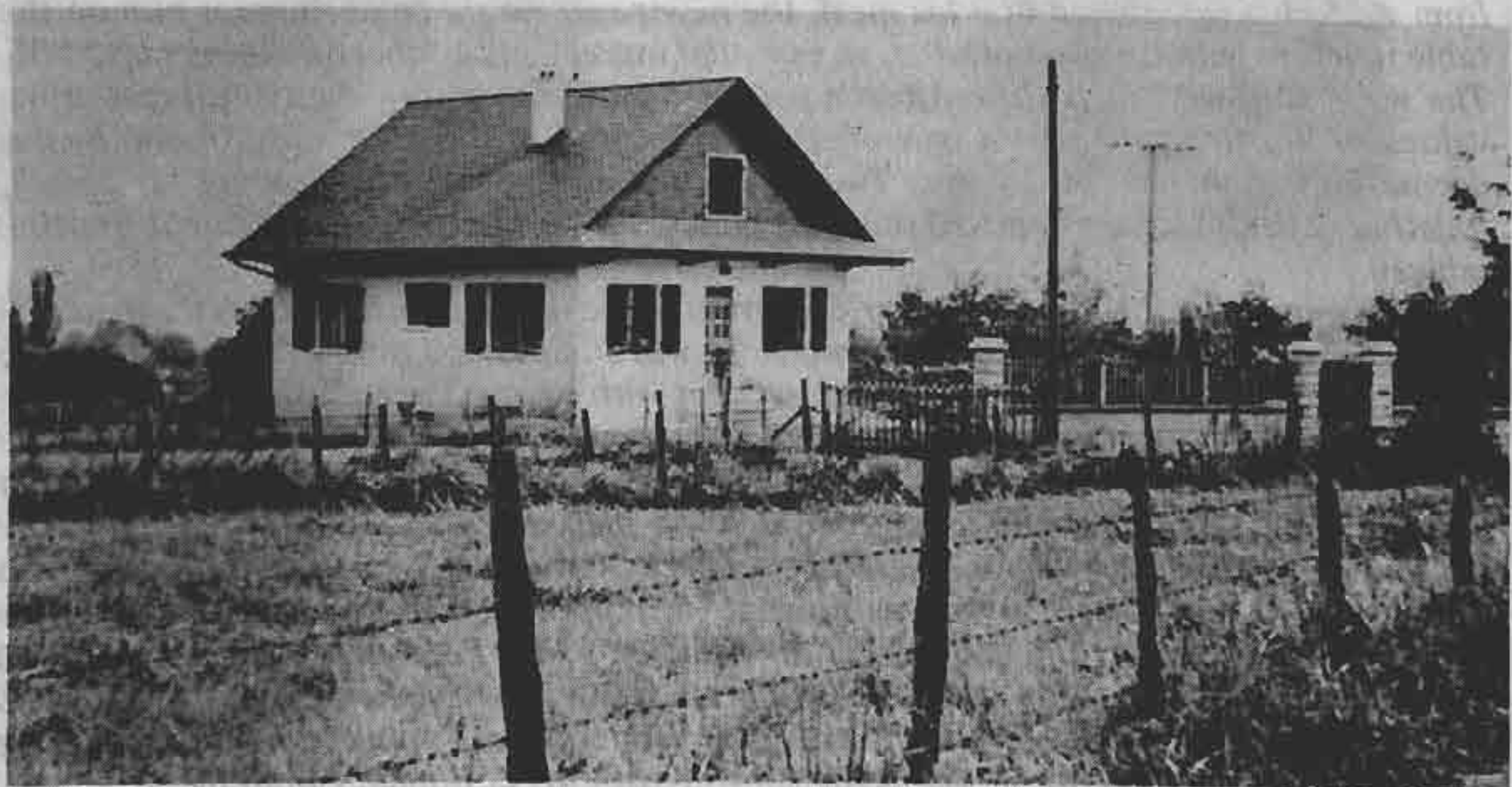
FIGURE 51: MR. HUGUET'S RAMMED EARTH HOUSE
