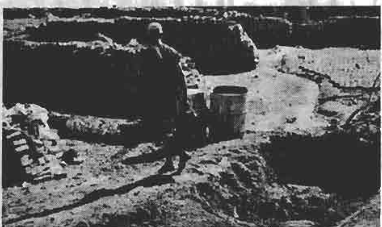
FIGURE 155: THE EARTH IS SHAPED INTO BALLS
