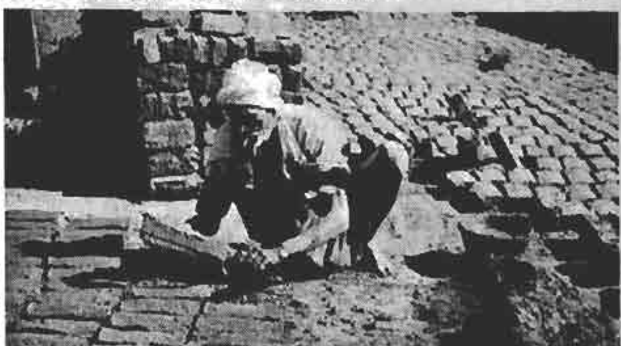
FIGURE 158: THE MOULD IS REMOVED AND THE PROCESS IS REPEATED.
