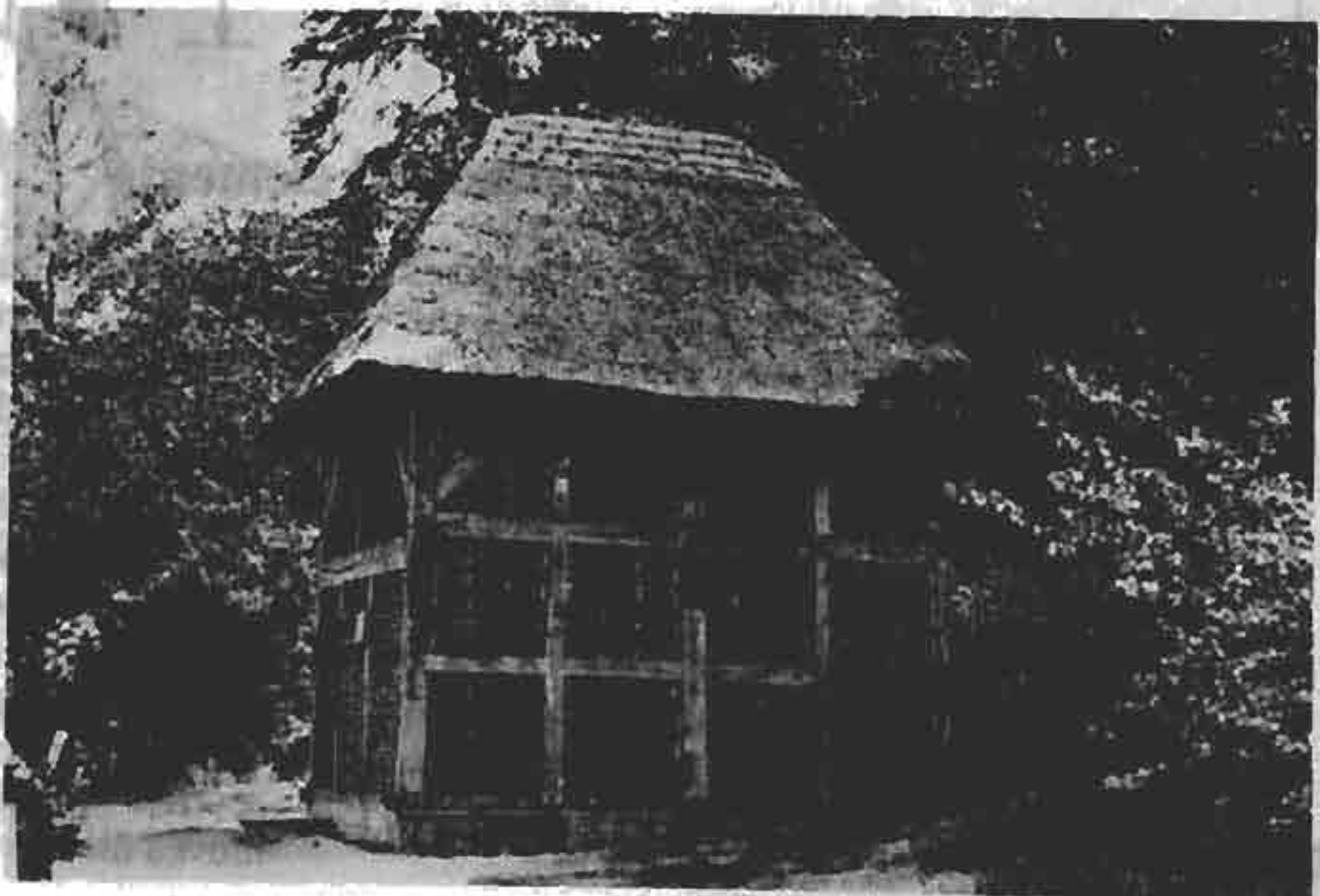
► FIGURE 293: CATHERINGTON TREAD WHEEL, 17TH CENTURY (SINGLETON OPEN AIR MUSEUM, ENGLAND). THIS LITTLE HOUSE SHELTERS A WHEEL WHICH MAY HAVE BEEN DRIVEN BY A MAN WALKING INSIDE IT TO RAISE WATER FROM A WELL. THE INFILL HAS NEVER BEEN PLASTERED, WHICH WAS NOT UNCOMMON AT THE TIME.
