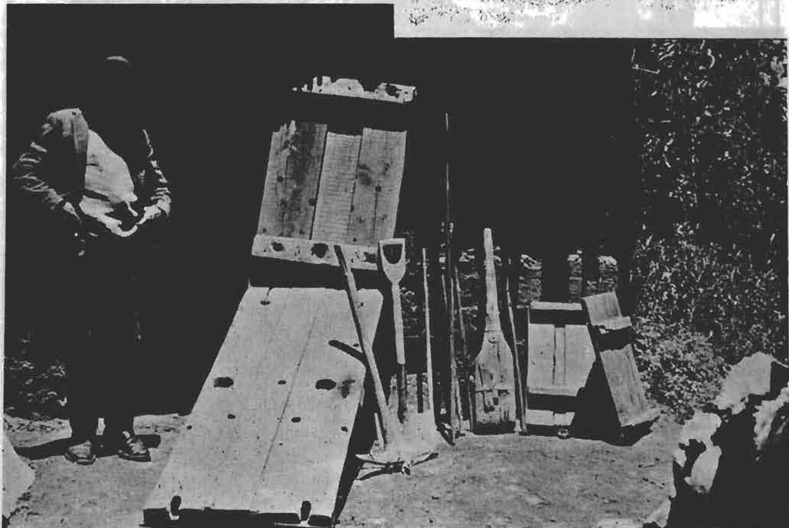
FIGURE 59: TOOLS USED FOR RAMMED EARTH IN PERU (HUANCAVELICA)
