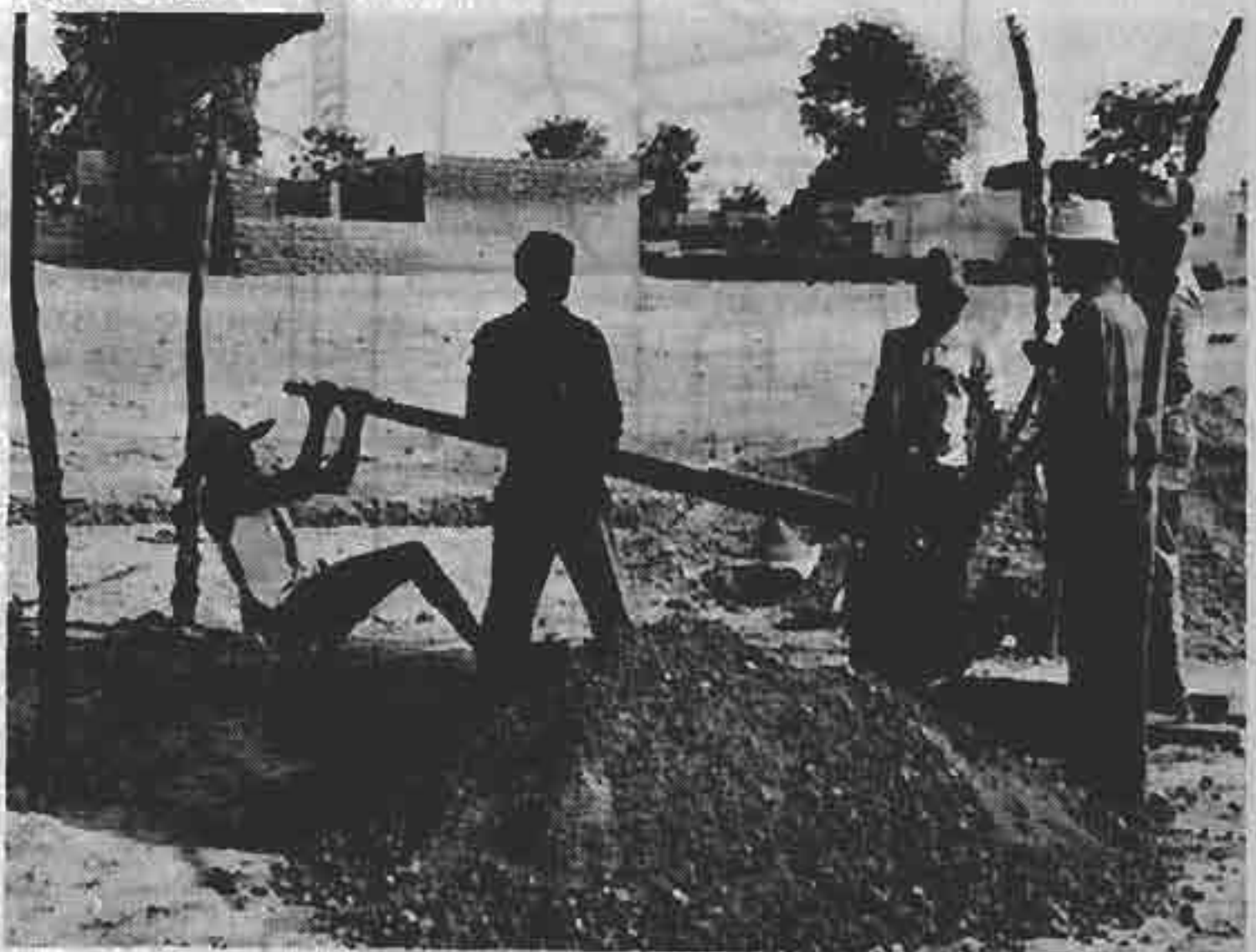
FIGURE 223: MAKING BRICKS WITH A TEK BLOCK PRESS (UPPER VOLTA)
