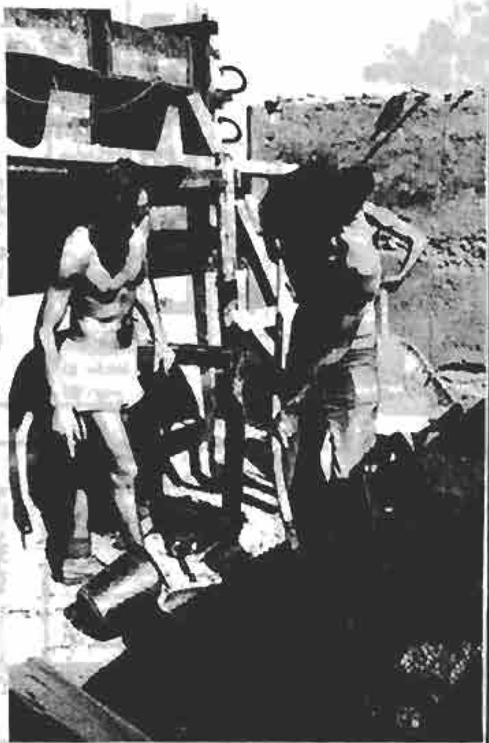
Mixing the earth and filling the formwork
