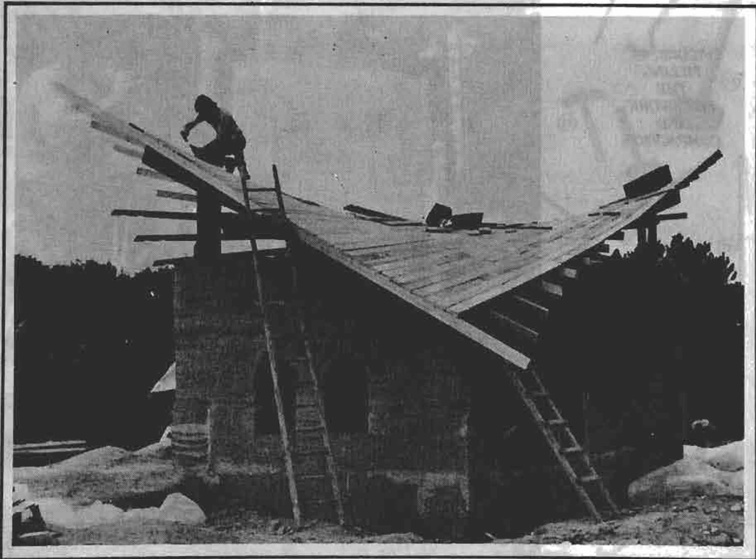
FIGURE 98: ON SITE AT VIGNIEU
