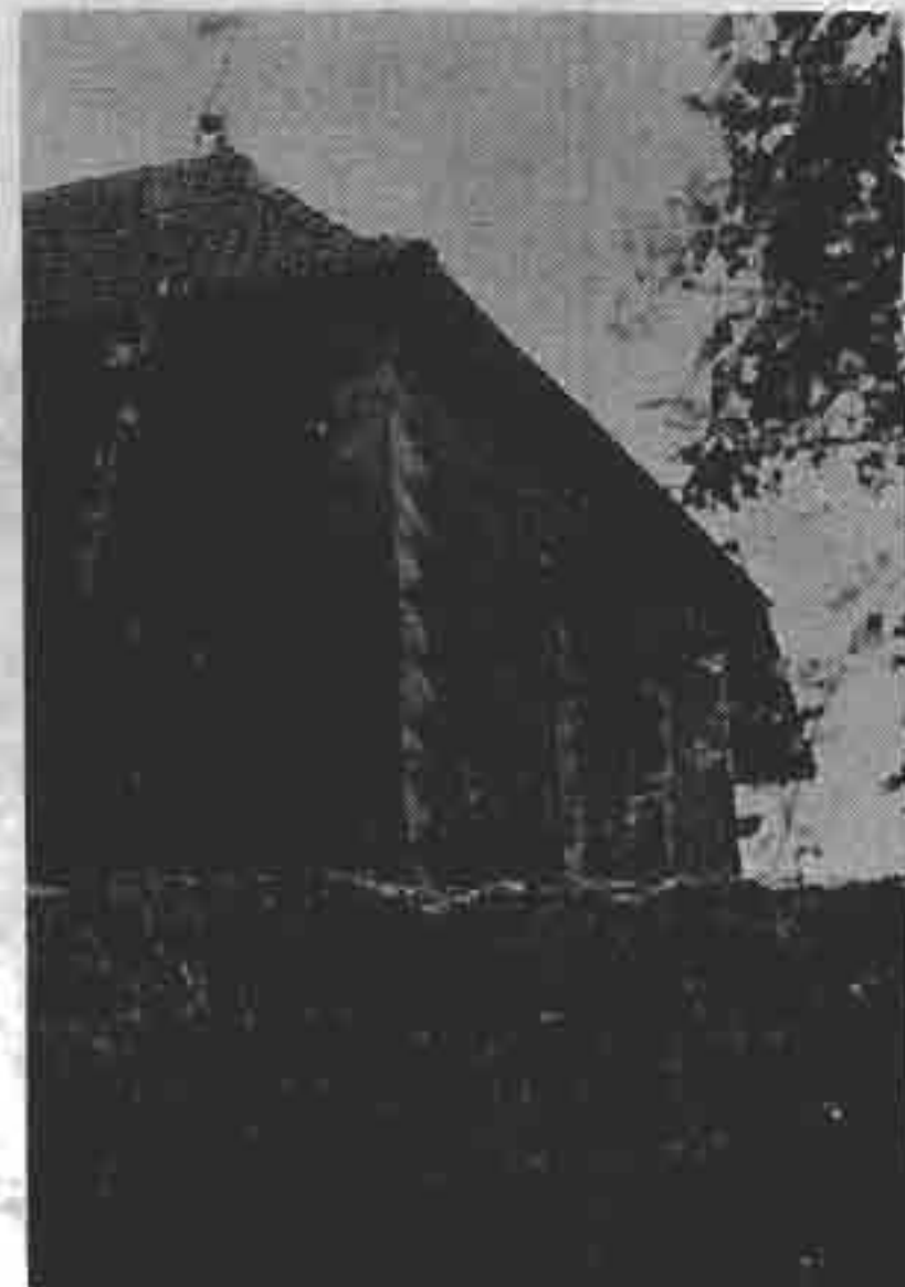
FIGURE 30: REINFORCING THE CORNER WITH "FLAGS" (ISERE, FRANCE).
