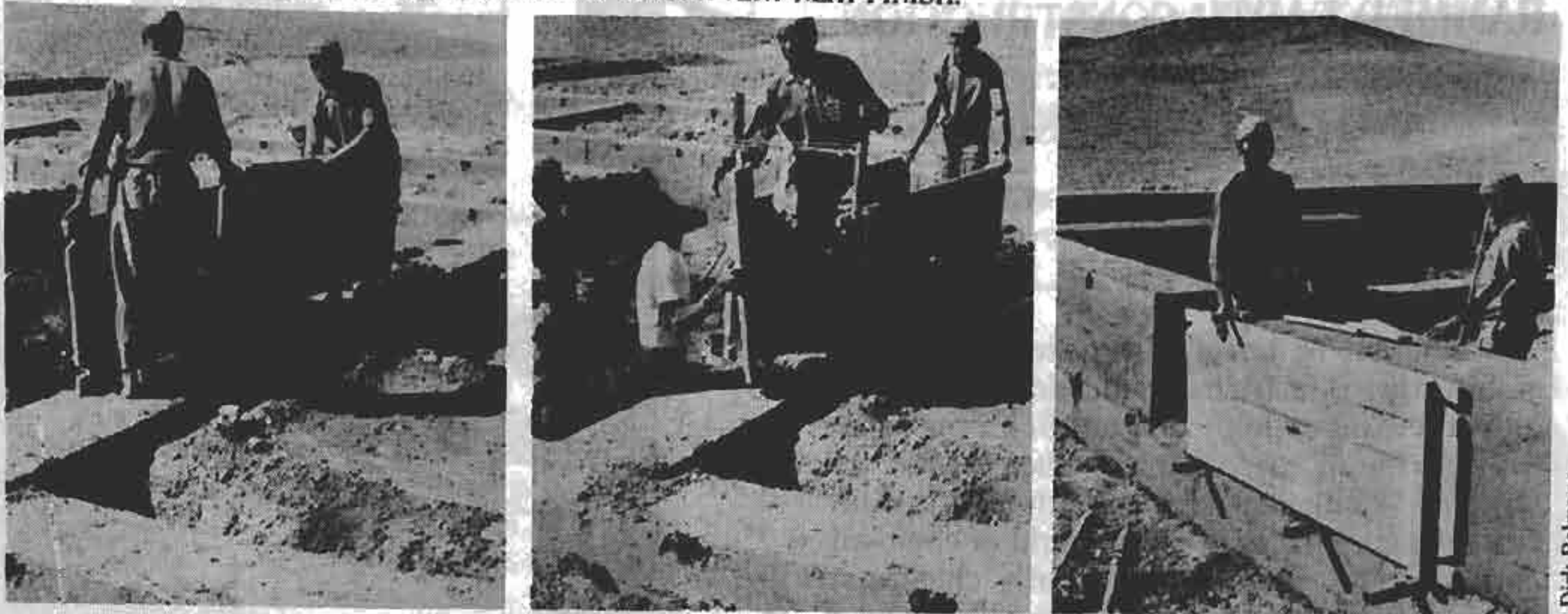
FIGURE 56: A REMARKABLY SIMPLE FORMWORK GIVES A VERY NEAT FINISH.
