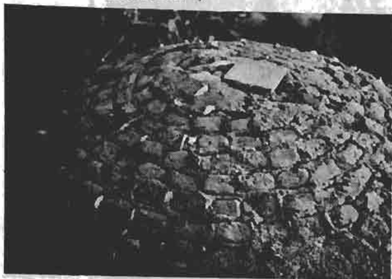
FIGURE 321: DOME BUILT WITHOUT SHUTTERING IN NEW GOURNA (EGYPT)
