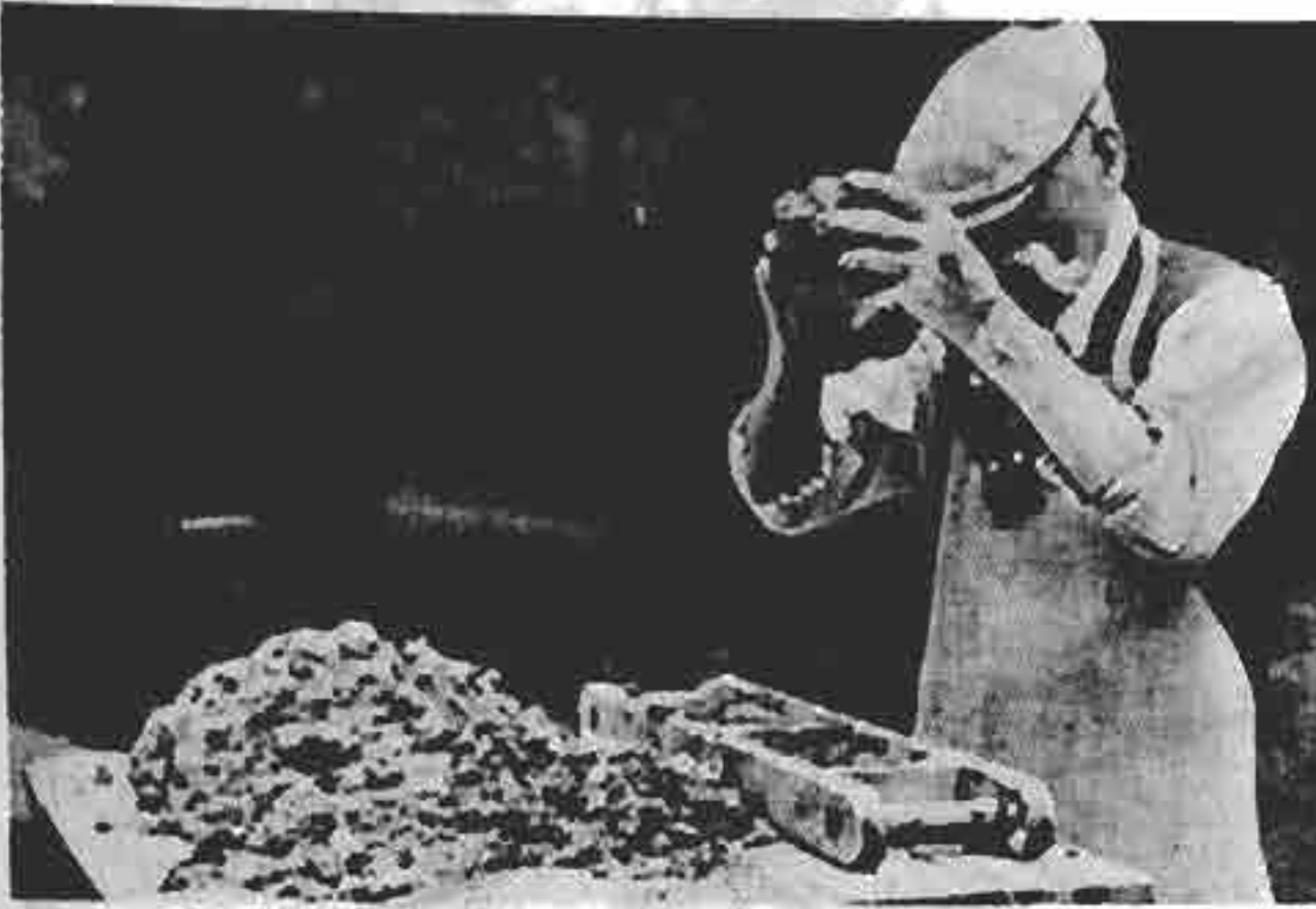
FIGURE 167: "BALL" MOULDING ON A WORK-BENCH (EAST GERMANY)
