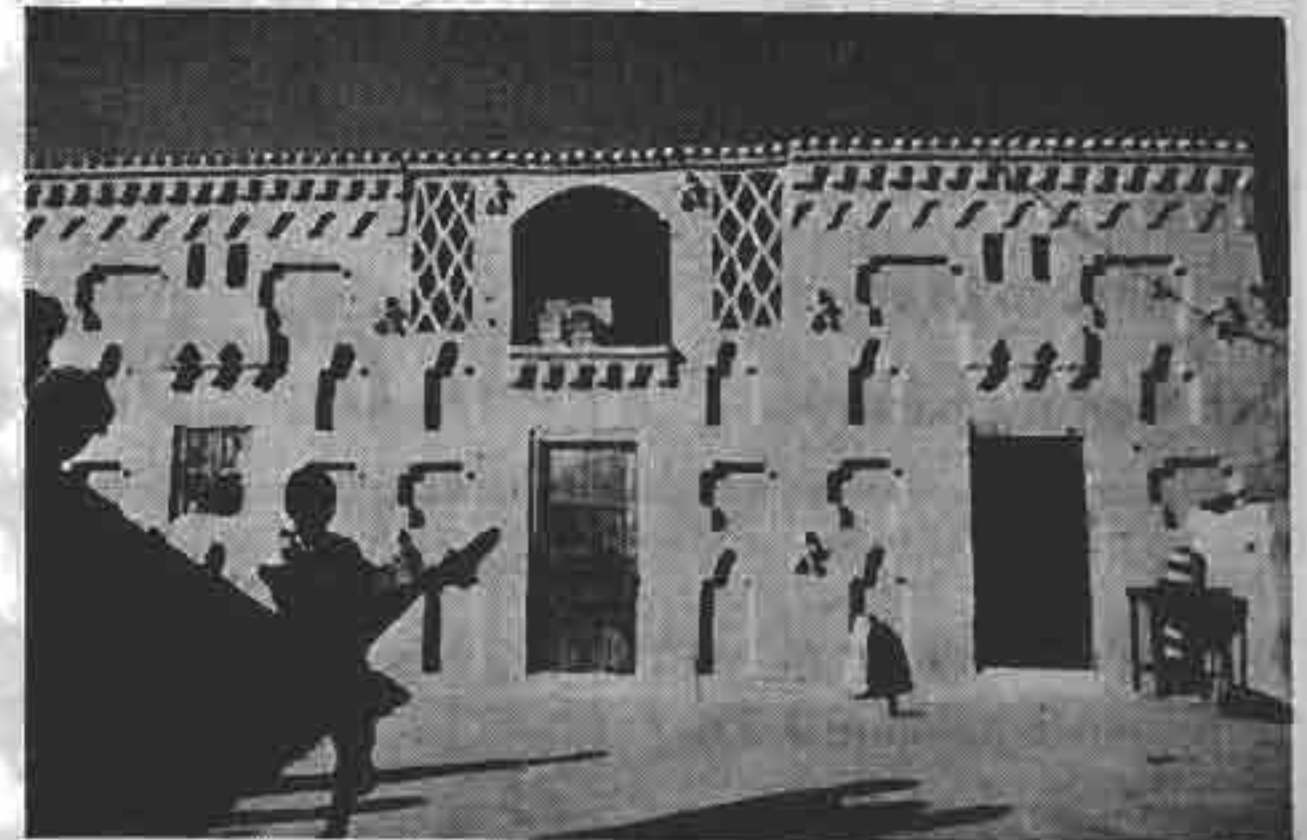
FIGURE 187: NUBIAN HOUSE NEAR ASWAN (EGYPT). THE DECORATIONS AND RENDERS OF THE FACADE ARE OFTEN DONE BY WOMEN.
