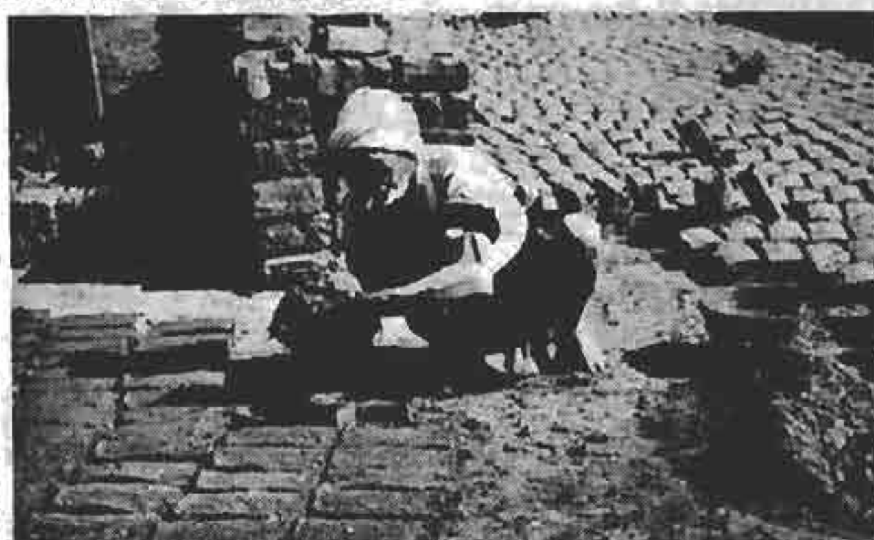
FIGURE 156: THE BALL IS WET BEFORE BEING THROWN INTO THE MOULD.
