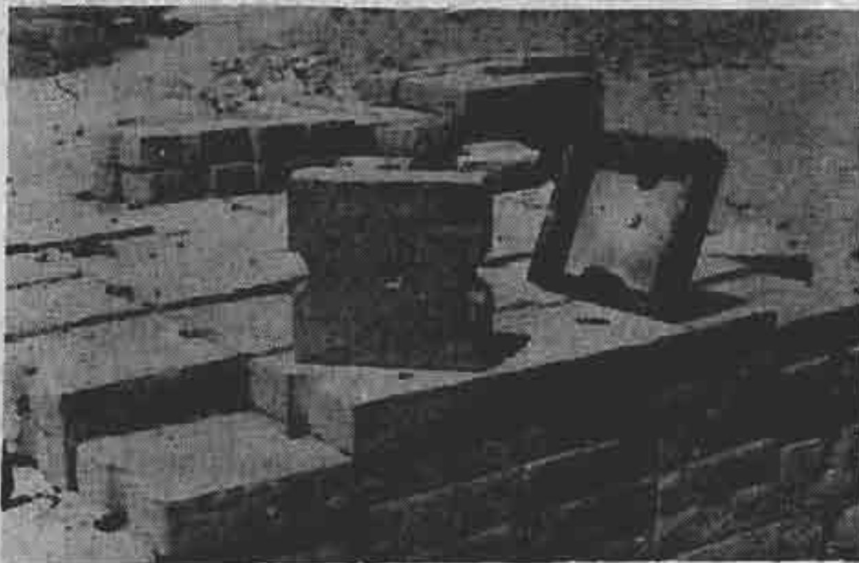
FIGURE 211: MOULD AND BRICK (EXPERIMENTAL HOUSE, LIMA).
